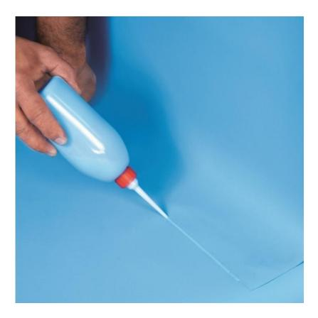
Apply liquid PVC in all areas where a weld was made to reduce the relief of the superposition of the membranes and to give greater sealing to the weld
