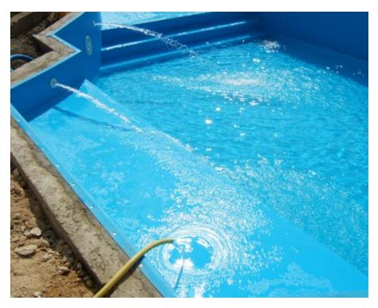
• This type of wall installation is done by making holes in the concrete and inserting stainless steel rivets to fix the membrane to the wall
